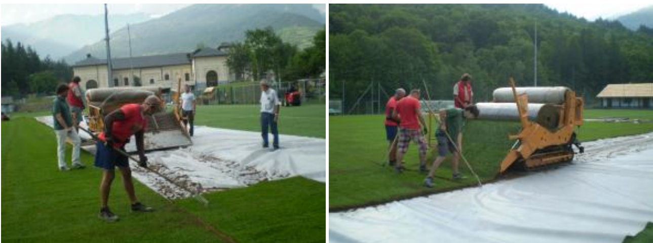
Applying the natural turf upon DuPont™ Typar® geosynthetics; photos by Bruno Marabotto, all rights reserved.
