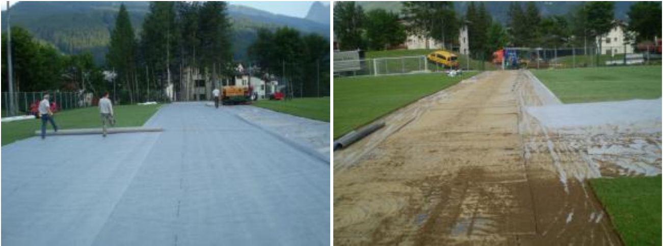
Installation of DuPont™ Typar® on the ground of Bardonecchia's football field; photos by Bruno Marabotto, all rights reserved.
